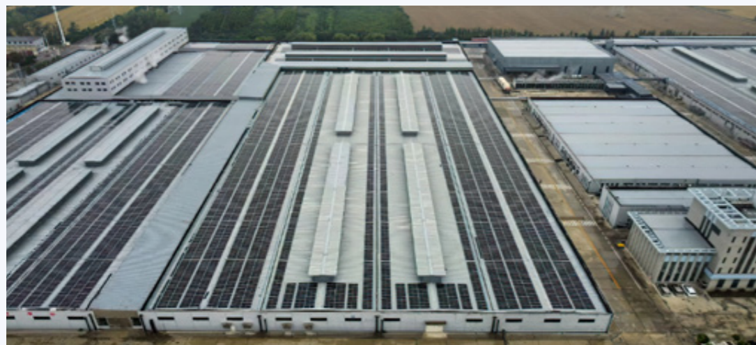
Photovoltaic Power Station in Zhende's Factory
